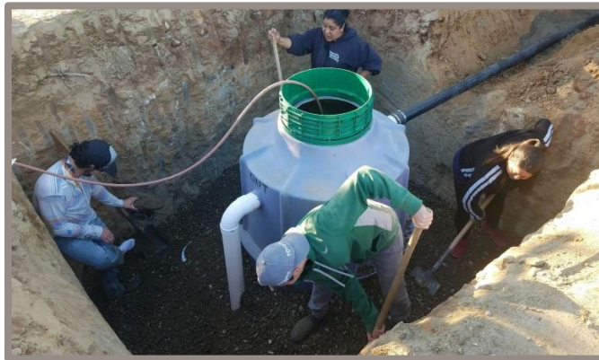
Septic tank molds (made by Dan Ouweleen's company, Pacmin) for Yorba Linda for Corazon house builds in Tecate, Mexico
